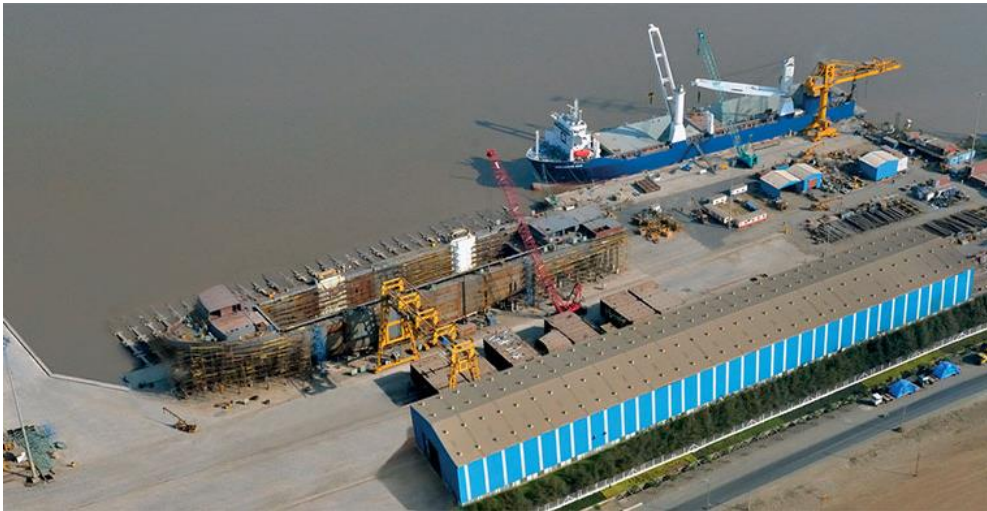
L&T Ship Manufacturing at Hazira
