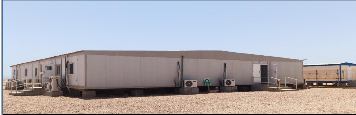
Site Office with Gravel Filling, Window ACs
