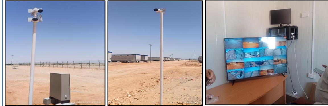
CCTVs & DVR Installation
