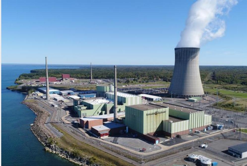
Nation's first integrated (behind the meter) 1.25MW PEM electrolyzer at a nuclear plant (Constellation)
